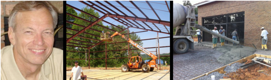
Reverend Henning and the work in progress
